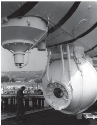
Figure I-1 - The Bathyscaphe Trieste, a work of engineering art and science, built by Auguste Piccard to mankind exploration of the deep seas. The Bathyscaphe Trieste was essentially a balloon which Piccard referred to as a float. The float consisted of a thin metal shell that was filled with gasoline, which would allow the float to ascend or climb in the water, once ballast was released. The two-member crew stayed in the observation gondola, a separate pressure sphere located at the bottom of the float. Source: U.S. Naval Historical Center Photograph, San Diego, California, 1958-59.
