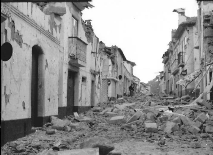
1980- Earthquake - Terceira, S. Jorge, Graciosa
