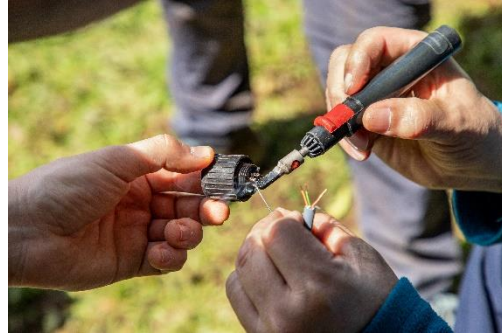
Photo B.30 - Welding connectors and cables.
