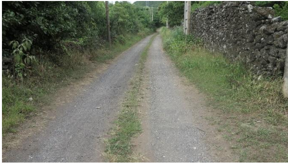
Photo B.44 - Road access.
