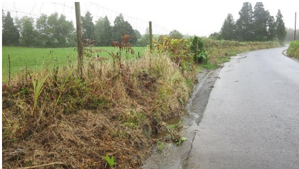
Photo B.102 - Road access and the result of 5 min lashing rain.
