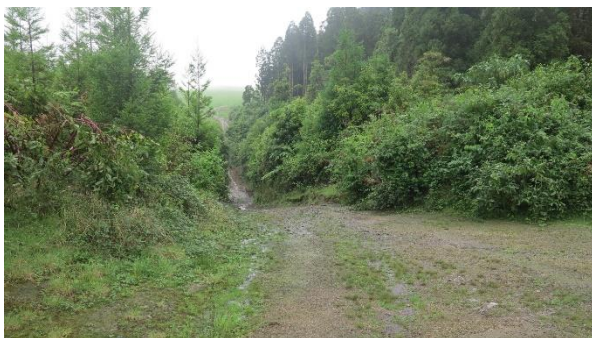
Photo B.104 - Impossible access to IS-FO-07_2 (on the right).
