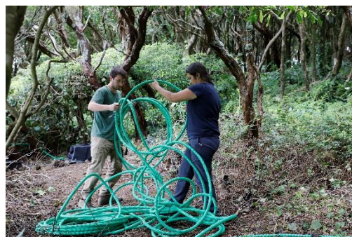
Photo B.28 - Extending electric cables already protected.
