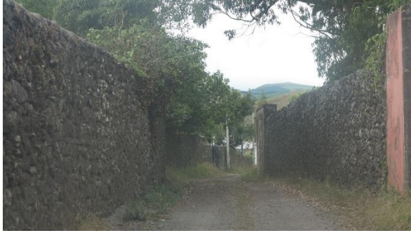
Photo B.50 - Walled dirt road to access IS-FO-02_2.
