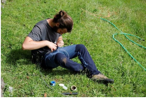
Photo B.29 - Welding connectors and cables.
