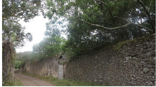
Photo B.51 - Entrance to IS-FO-02_2 closed.
