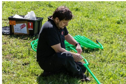
Photo B.26 - Preparing protection tubes to insulate electric cables.
