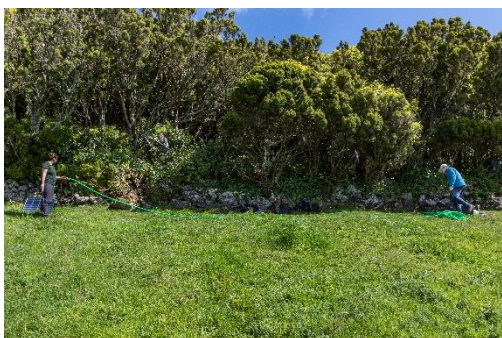
Photo B.27 - Preparing protection tubes to insulate electric cables.
