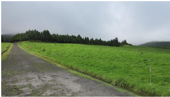
Photo B.86 - Road access (forest at the back).
