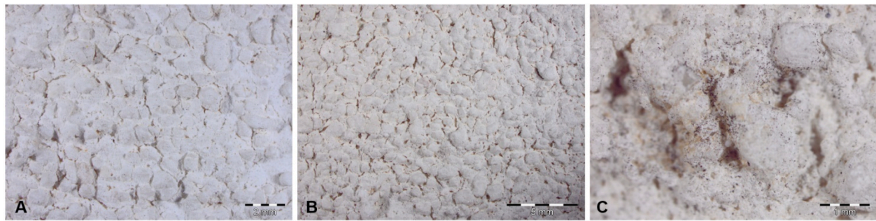
Fig. 6. Microcracking observed on the surface of the artificially aged (A) and 3-months naturally aged system S2 (B); dirt deposition on the surface of the naturally aged system S3 after 9 months of outdoor exposure facing North (C).
