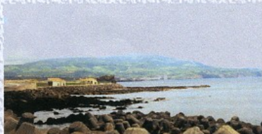
Fig. 1. General view of the Wastewater Treatment Plant
